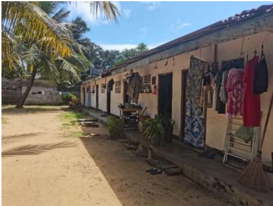
Figure 1: Line rooms at the front entrance of a boarding house
